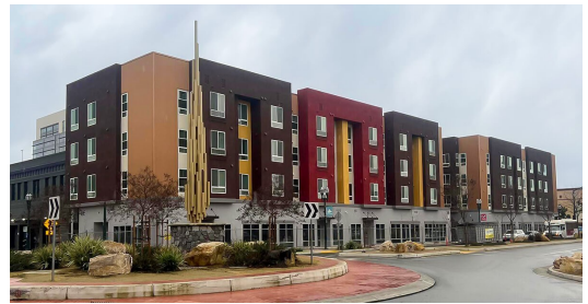
Grand View Village on Minor Ave, Stockton
